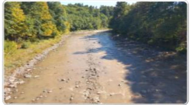
Photo of Esopus Creek Below Five Arch Bridge on October 11, 2016.
